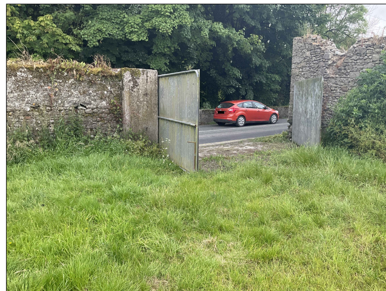
PHOTO OF EXISTING ACCESS GATE FROM R693 TO PRIVATE LANDS.
