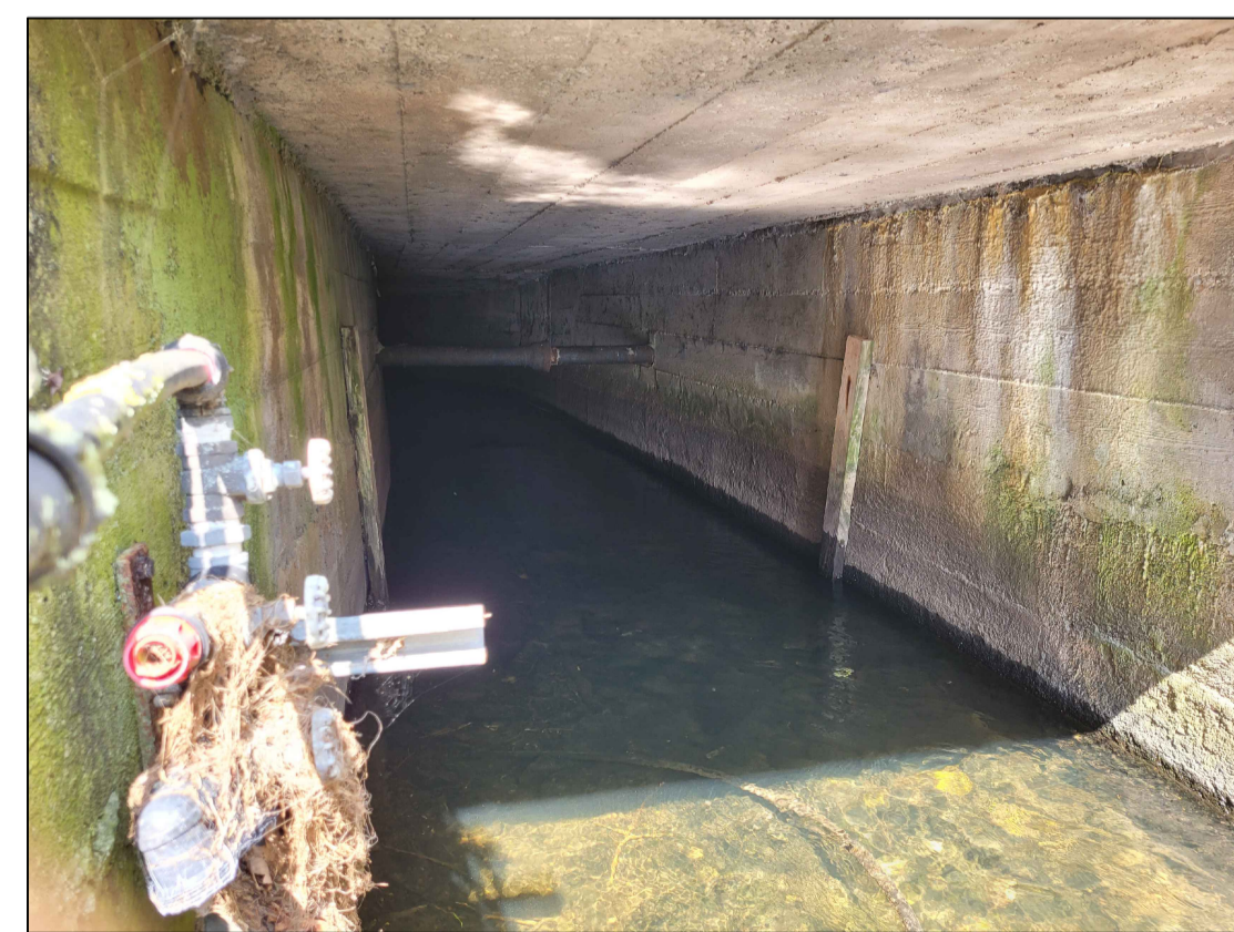
PHOTO OF 2 SPAN BRIDGE CULVERT
