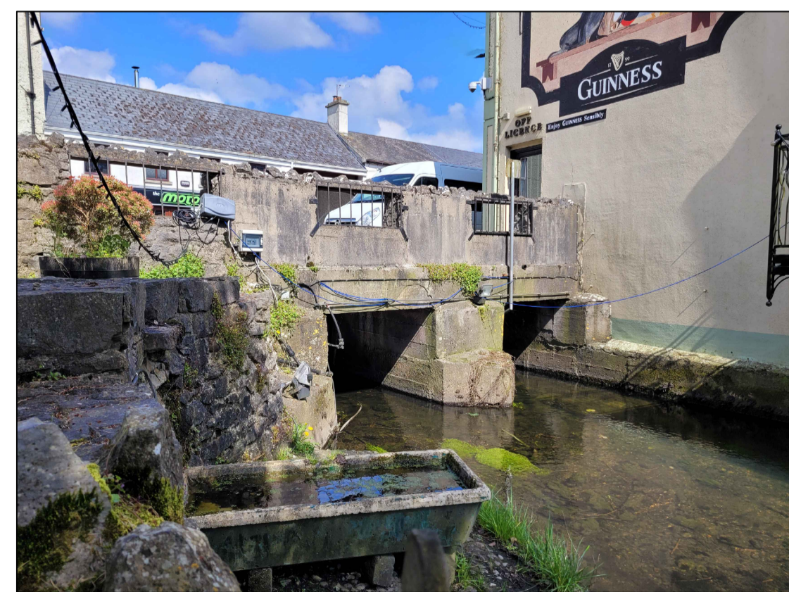
PHOTO OF 2 SPAN BRIDGE CULVERT
