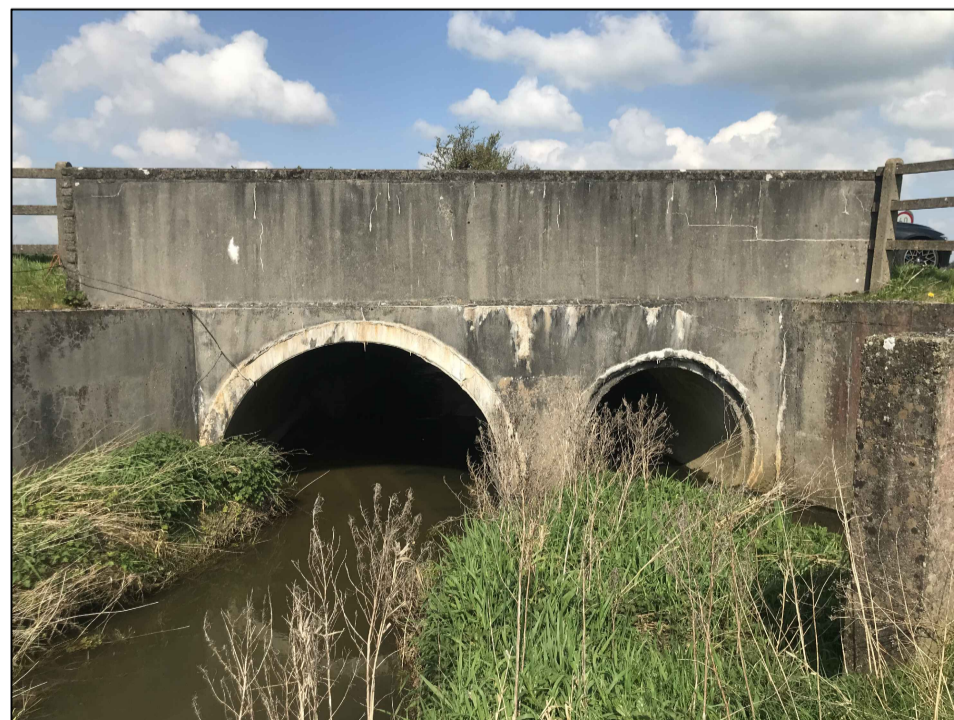
PHOTO OF 2 LARGE DIAMETER CULVERTS ON GOUL RIVER
