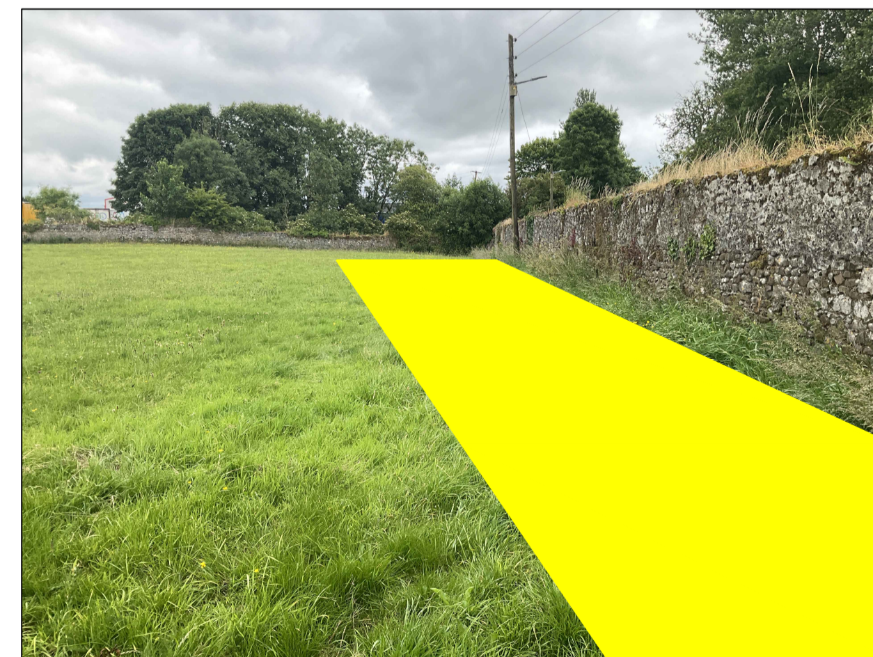
PROPOSED 5m WIDE WAYLEAVE TO FACILITATE ACCESS ROAD TO RUN TIGHT AGAINST EXISTING BOUNDARY WALL & STOPPING AT HDD LAUNCH PIT LOCATION.
