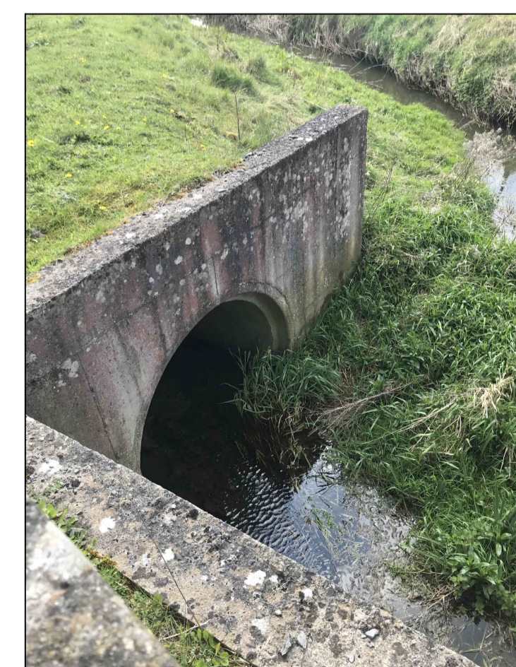
PHOTO OF 2 LARGE DIAMETER CULVERTS ON GOUL RIVER
