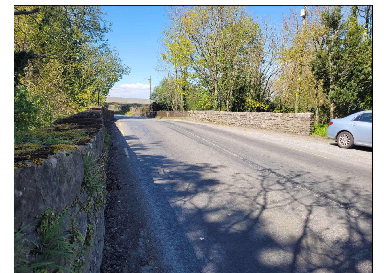
PHOTO OF VIEW FROM R693 TOWARDS THE SINGLE ARCH BRIDGE
