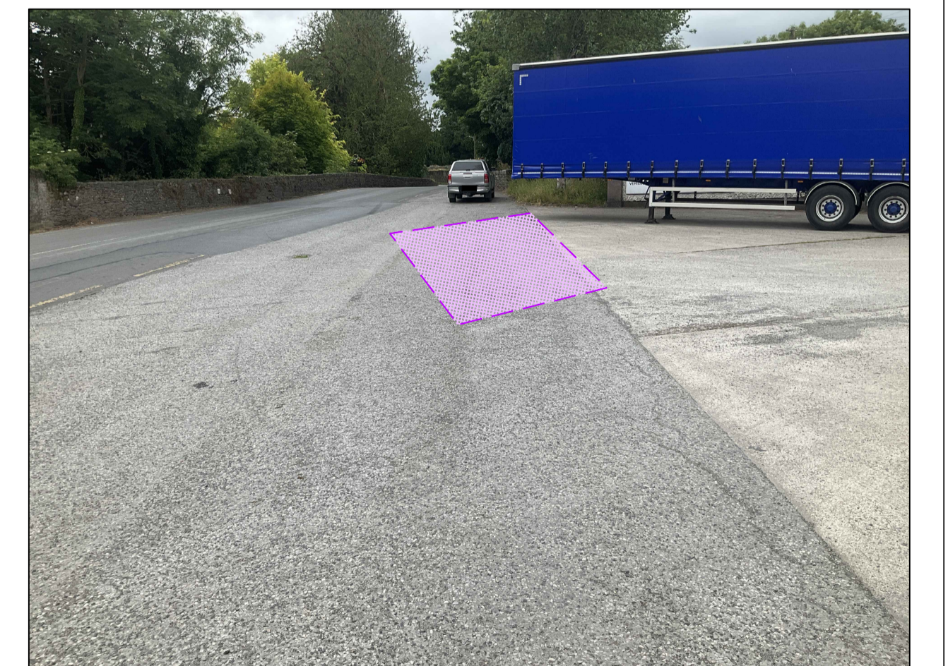
PROPOSED HDD EXIT PIT TO BE LOCATED WITHIN VEHICLE TESTING CENTER ENTRANCE.
